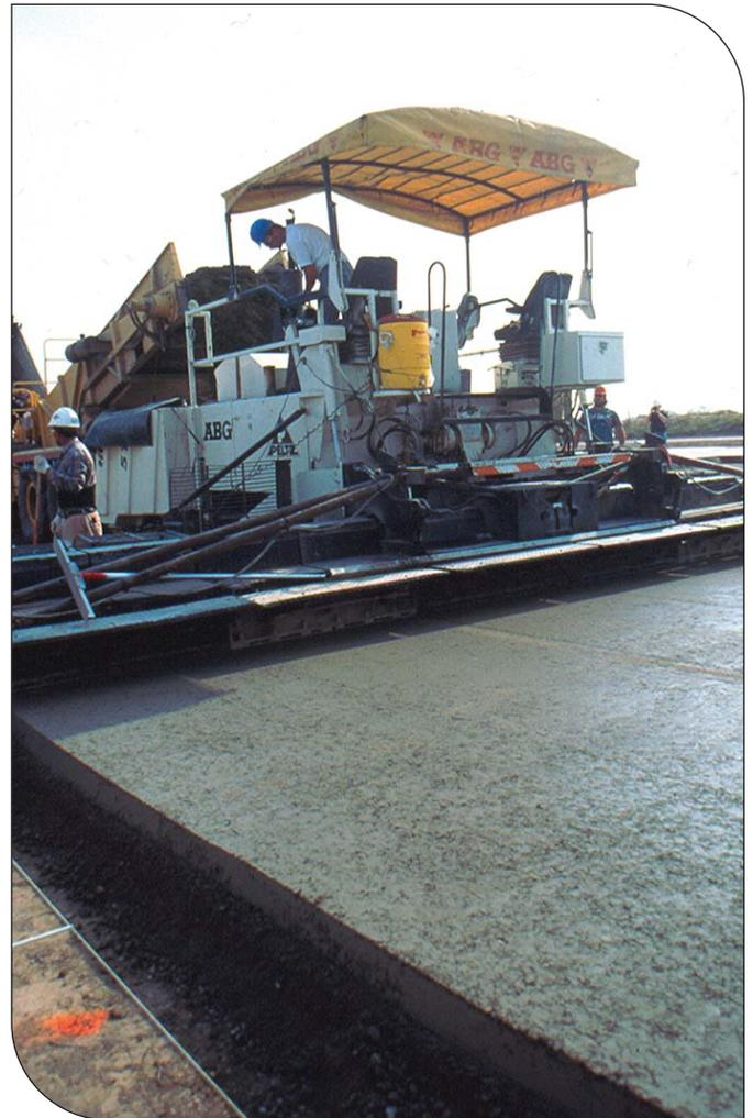
**RCC normally is placed with asphalt paving machines; most contractors who specialize in the construction of RCC pavements use high-density pavers with vibrating screeds and oscillating tamping bars.**
