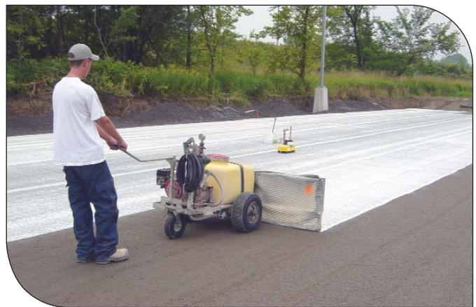
**A key to long term performance is adequate curing. Water or concrete curing compounds are typically used.**
