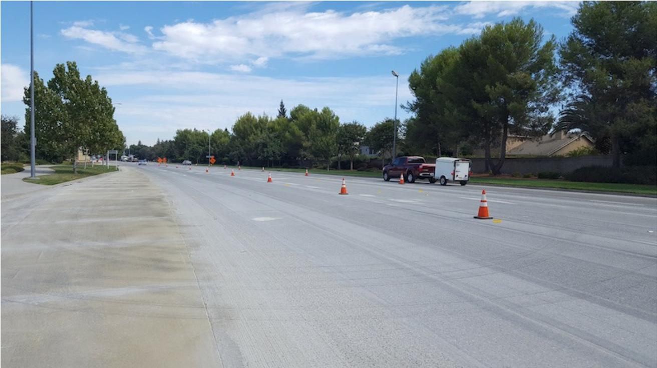
Roller-compacted concrete pavement after diamond grinding. Photo courtesy: Corey J. Zollinger.
