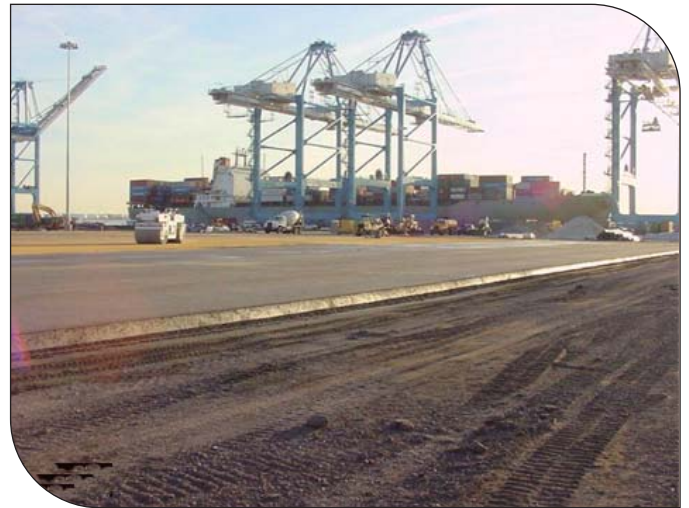
Completed RCC slab.
