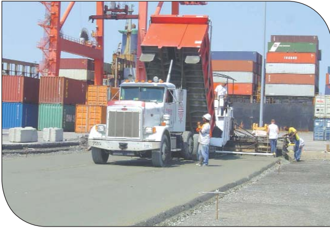
Paving top lift within 1 hour of bottom lift placement.
