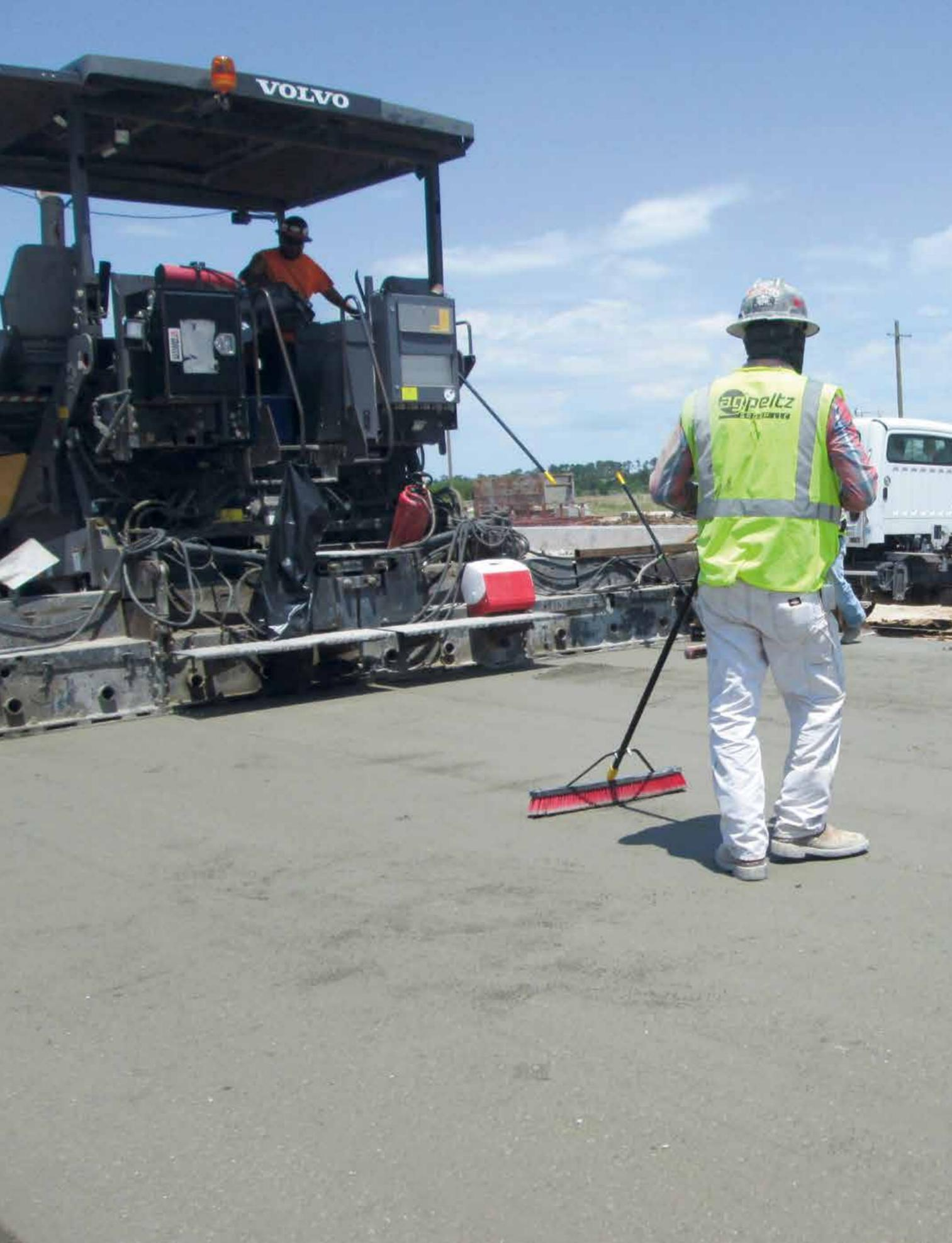
Cost-effective and durable, roller-compacted concrete (RCC) pavement is laying a solid foundation for a number of significant projects for the Port of Houston Authority (PHA). By 2020, the Port is expected to have 380 acres of mostly 18-inch-thick RCC, making it the largest RCC site in the U.S. For perspective, a similar amount of RCC would fill a 6-inch-thick single lane road stretching more than 800 miles across Texas from Orange to El Paso.
