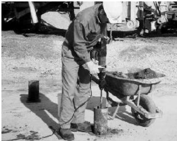
Figure 2. The vibrating hammer in the field (provided by PCA).
