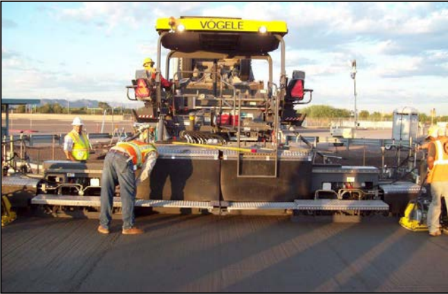
Figure 8. High-density RCC paver.
