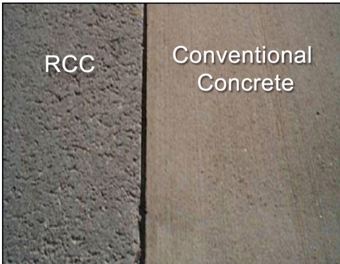
Figure 5. RCC surface texture.
