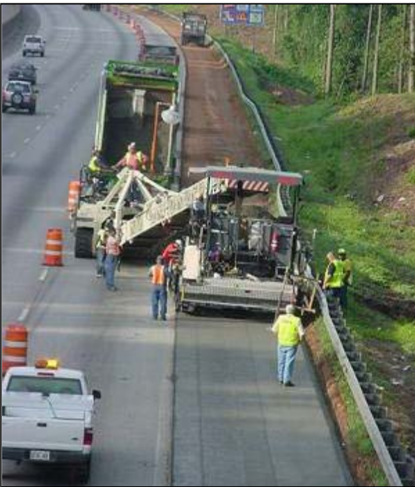
Figure 9. RCC construction.
