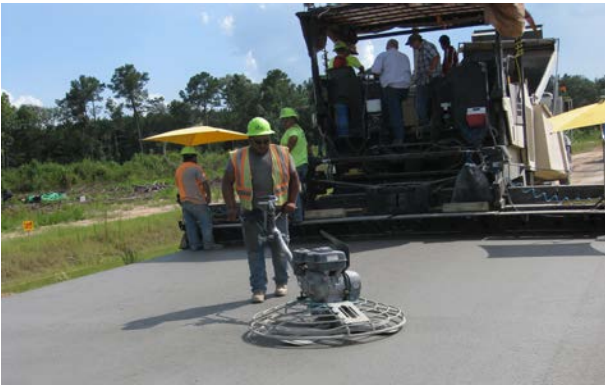
Figure 12. Method to improve upon RCC finished surface.
