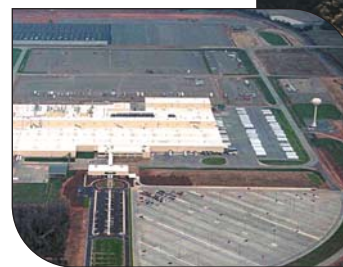
Approximately one million square yards of RCC pavement was placed at the Honda plant in Lincoln, Ala.
