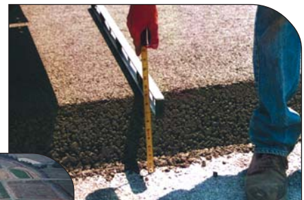
At the Mercedes-Benz auto plant in Vance, Ala., a pavement engineer measures the depth of the placed RCC.
